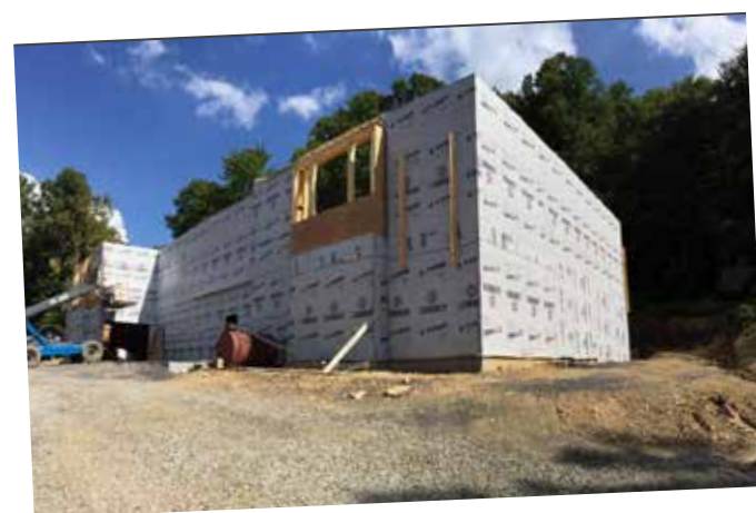
New school under construction.
